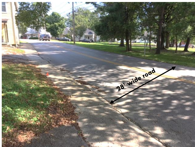
PHOTO 1: Northern View of Winchester St.
