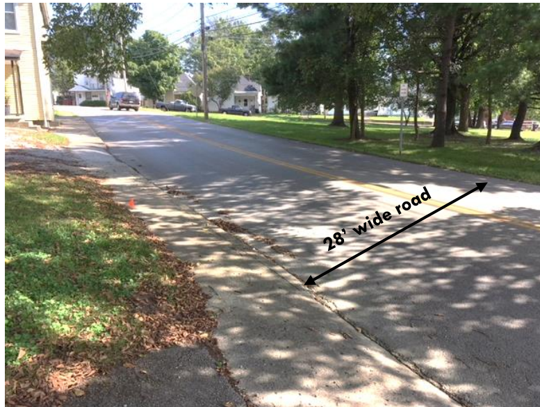
PHOTO 1: Northern View of Winchester St.
