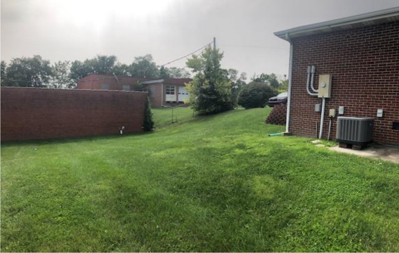
Southern view of building toward "Bud's Gun Shop". French drain proposed to contain and redirect runoff from the next addition to prevent it from entering the adjacent property.
