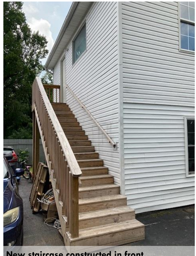
New staircase constructed in front.
