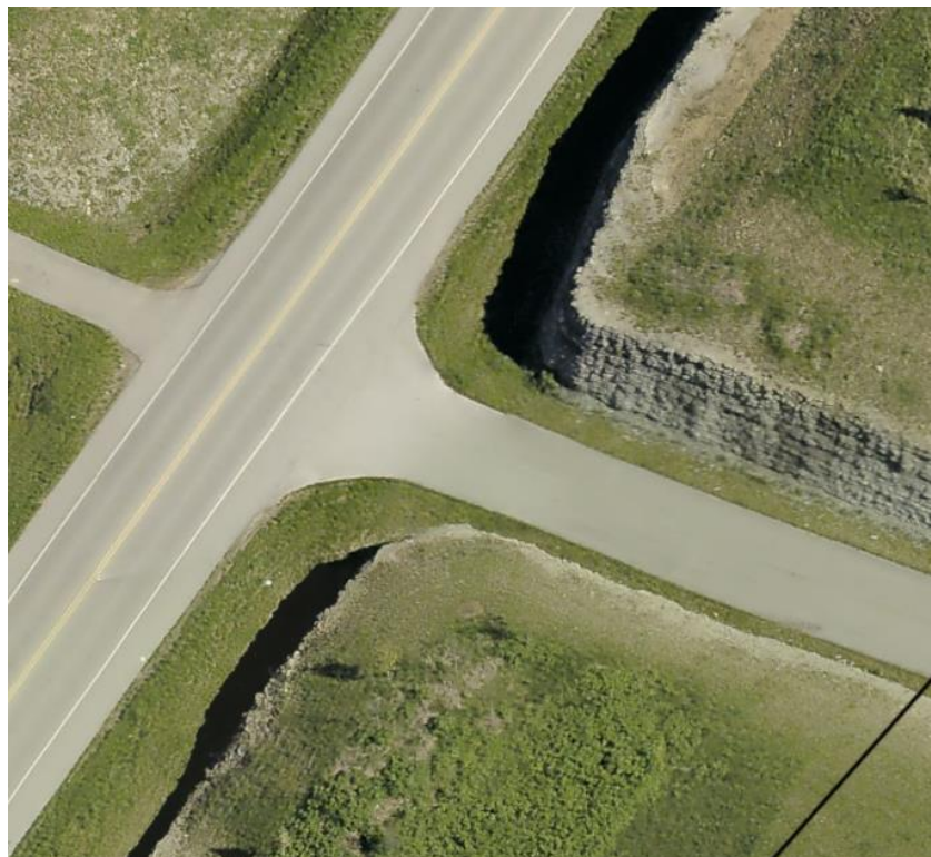
US 68 Entrance Aerial View
