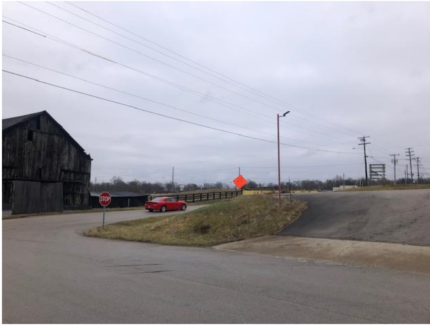
View of intersection of Wes-Lee and Fords Mill Rd. Entrance to subject property shown on right hand side of photo. Note: Change in elevation from street grade to site)
