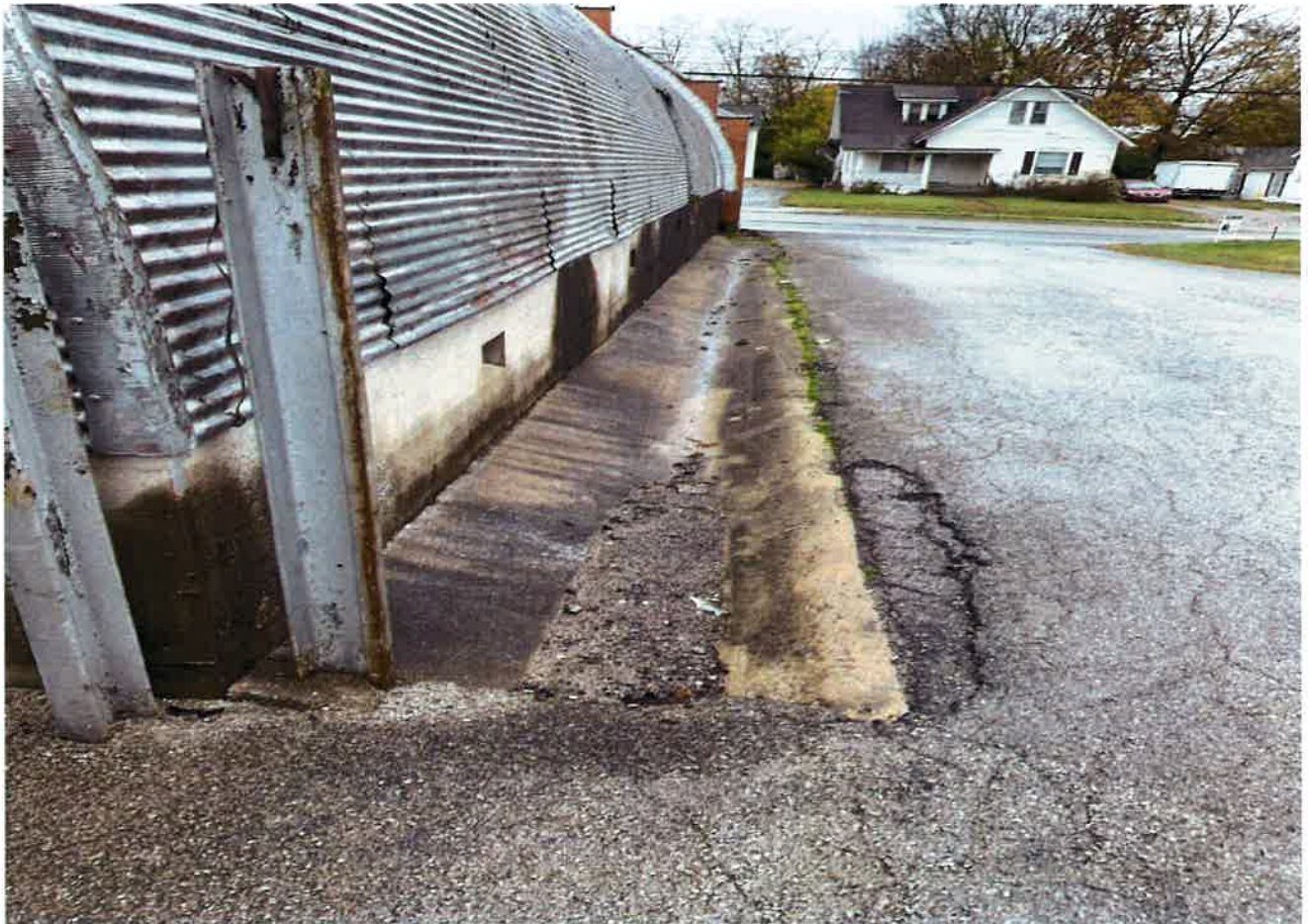
Paved ditch at North Exit on main street
