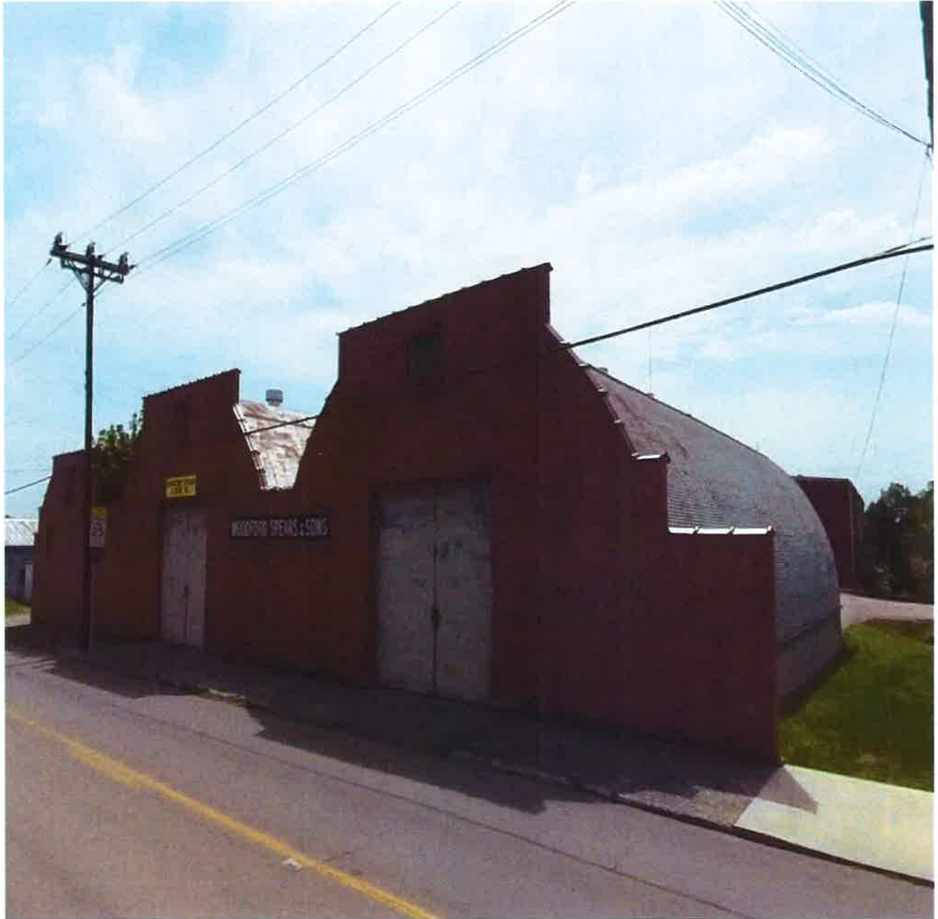
Quonset buildings – front (west view)
