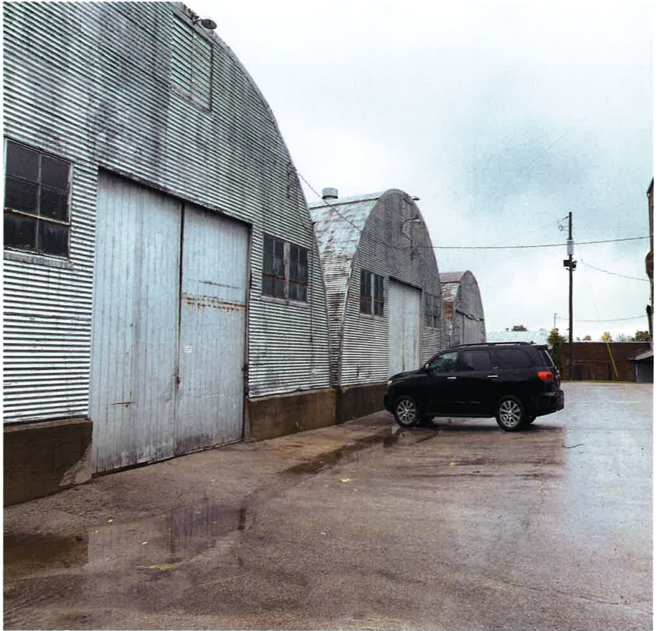
Quonset buildings – rear (east view)
