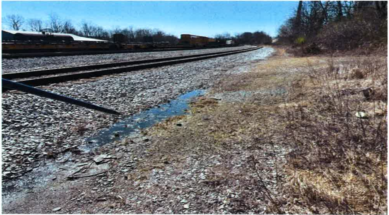
Drainage ditch -east side of property – looking south
