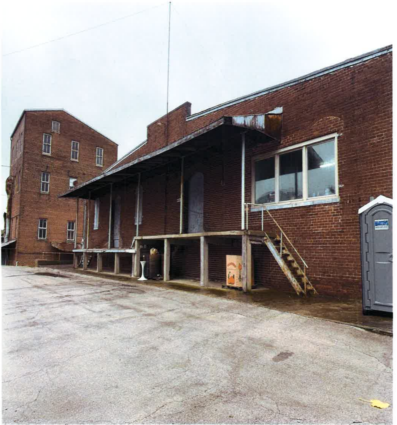
Existing Spears Office Building (foreground); Tower Building (background) west view
